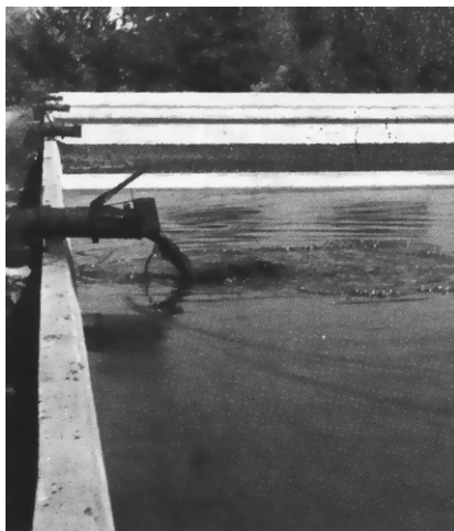
Solids suspended in water are pumped into a sludge field.
